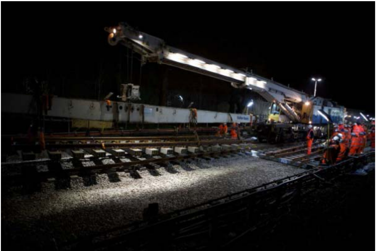
Modular points and crossings installation at Ruislip
