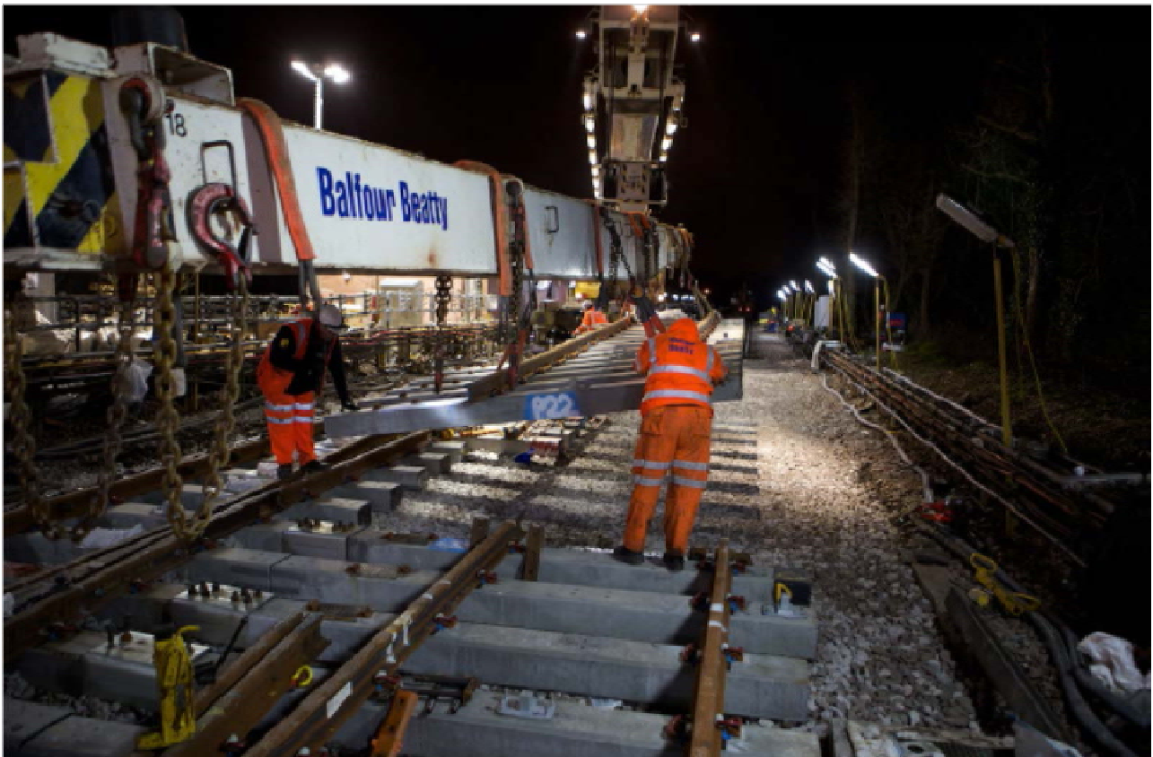
Modular points and crossings installation at Ruislip
