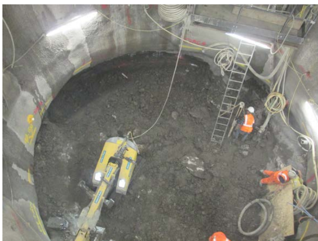
Vauxhall station shaft excavation
