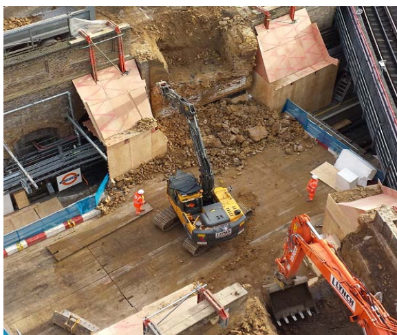
Whitechapel Station Winthrop St bridge removal
