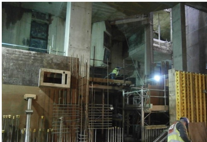
Fixing and pouring walls in the LU station box at Bank station
