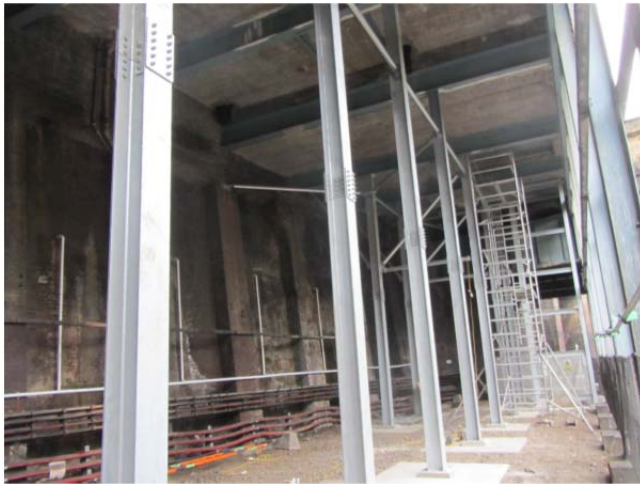
Floor strengthening steelwork as Farringdon
