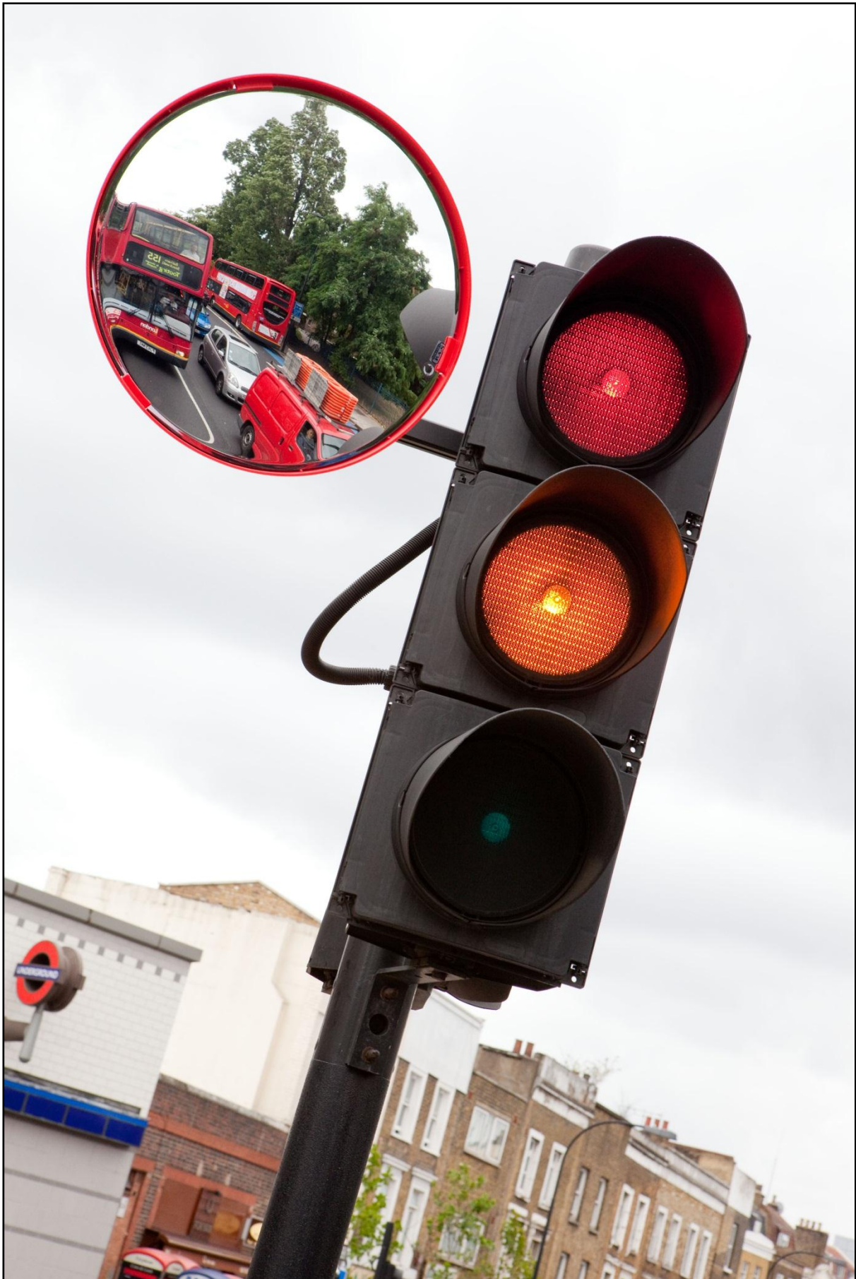
Converting traffic signals to LED extra low voltage
